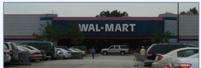
Existing Wal-Mart, located off of IL Route 83
